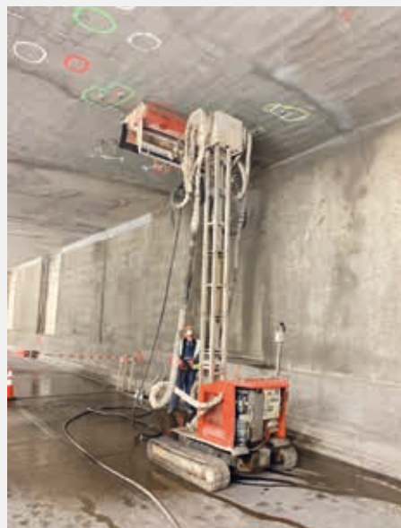
Tunnel Brussel – Hydrodemolition plafond op 4 cm.
