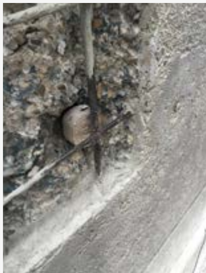
BP Building Galvashield2 close up
