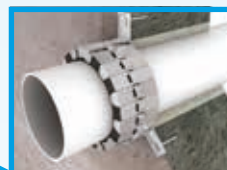
fire stopping en fire sealing
